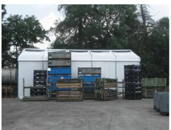
Due to a new contract, ARRK Europe needed a warehouse structure to serve as an additional storage facility. As such, J & J Carter installed a Series 170 10m x 12.5m with a side height of 4.4m. The structure was erected in just two and a half days.
