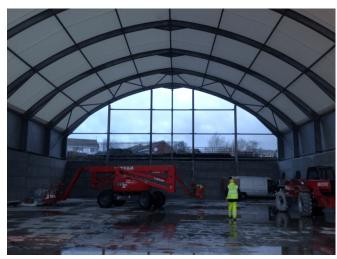
Rochdale Council required a Saltbarn to store 5000 tonnes road salt at their Princess Street Depot. J & J Carter were contracted by Kaberry Construction to design, manufacture and install the tensioned fabric roof membrane. J & J Carter also assisted with the detail design of the steel frame to resolve the fabric interfaces.
