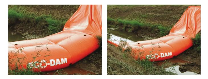
The EcoDam is being used as a cofferdam to hold back water. We also provided the anchorage system to hold the barrier either side of the ditch.
