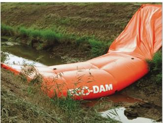
The EcoDam is being used as a cofferdam to hold back water. We also provided the anchorage system to hold the barrier either side of the ditch.
