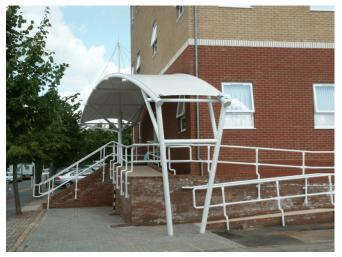
J & J. Carter Ltd were commissioned by the client to design and build a new canopy to the original scheme as designed by Sutton Griffiths. The new canopy has been built using a welded steel frame work, with stainless steel tension cables and a White PVDF lacquered PVC fabric.
