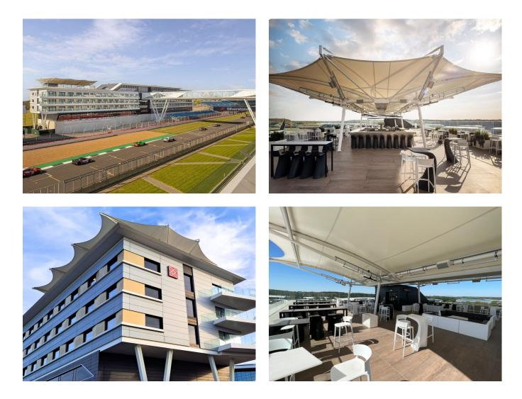
A new 197 bed Hilton Garden Inn Hotel has been built over looking Silverstone's iconic starting grid and pit lane, adjoining the racetrack. The 6-storey structure is built on a concrete frame on the ground and first floors with a lightweight steel frame upper section.
