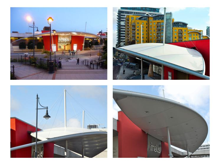
The Basingstoke improvement works included the installation of a clear roof canopy and removing heavy over-hanging concrete canopies.
