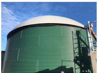
J & J Carter were contracted to design, manufacture and install a PVC membrane cover for an anaerobic digester used to produce biogas at Windover Farm in Hampshire.
